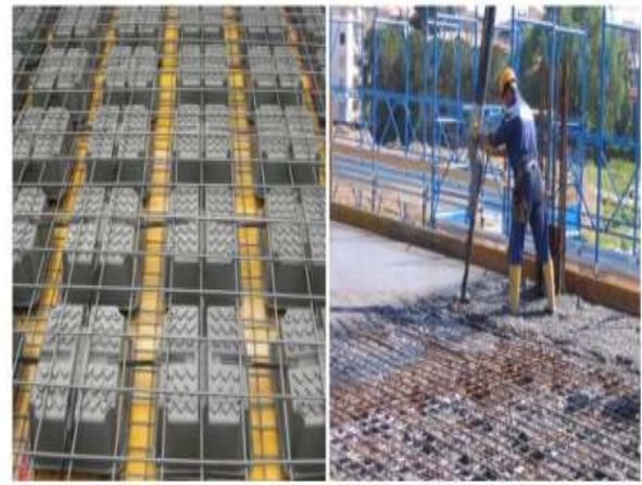
Fig.3 Installation of U-Boot Beton
