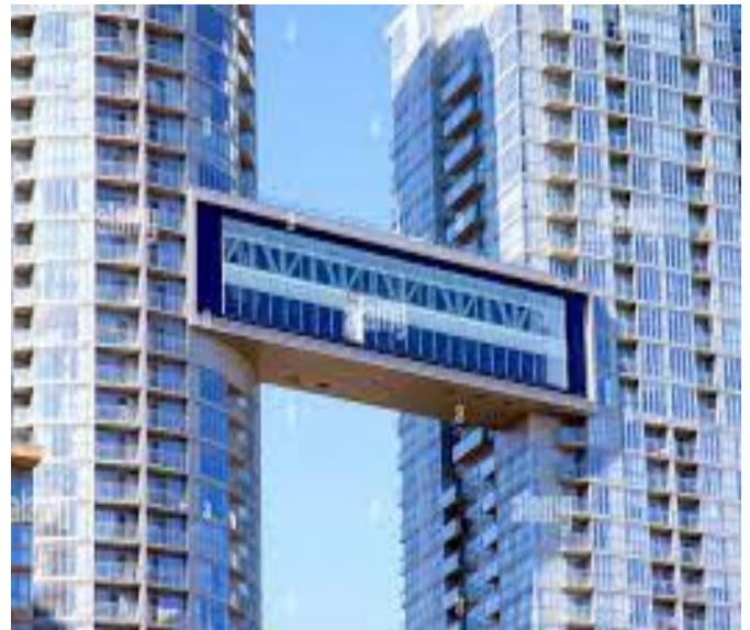
Fig. 3: Bridge connecting two condo buildings
